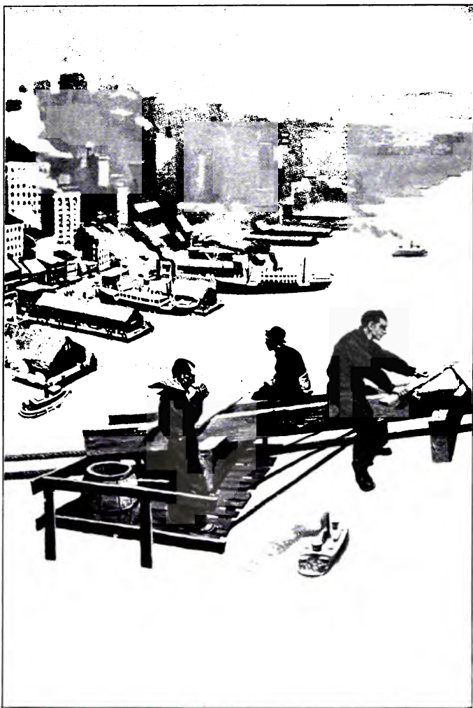
WITH THE TEMPORARY CABLES IN PLACE, THE WORKMEN BEGIN BUILDING A FOOT-PATH
